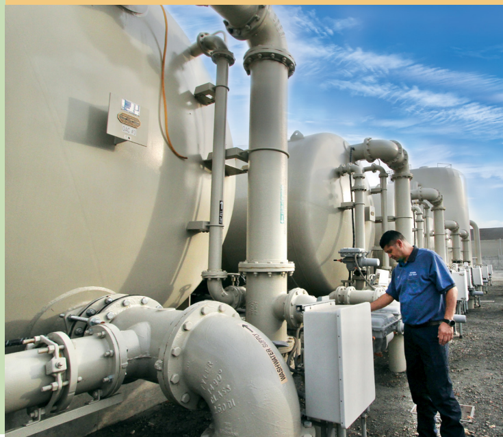
Surface water that originates as snow and rain in the Sierra Nevada range is treated at our local Lessalt and West Hills Water Treatment Plants, then blended with local well water. Shown here are Lessalt's activated carbon filters, which remove microscopic organic contaminants.
