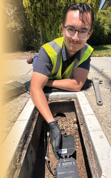
Jorge Mendoza installs a new radio read meter, which gives customers detailed online access to their water use data (see back page WaterSmart article).
