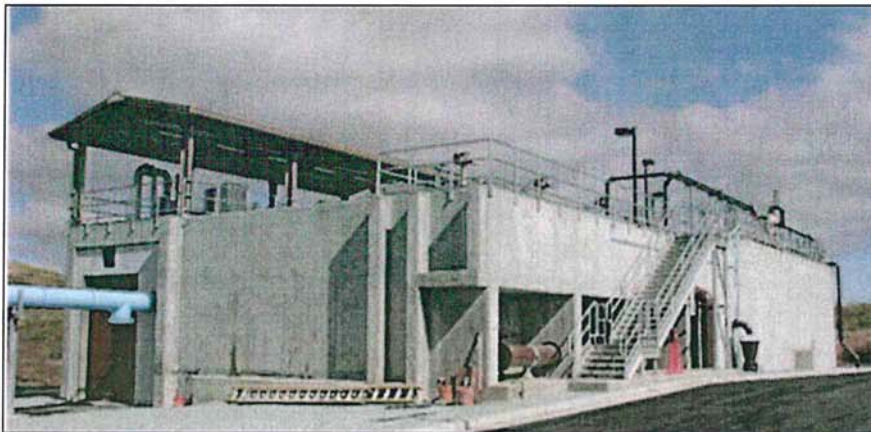
Figure 2-3. West Hills Water Treatment Plant
