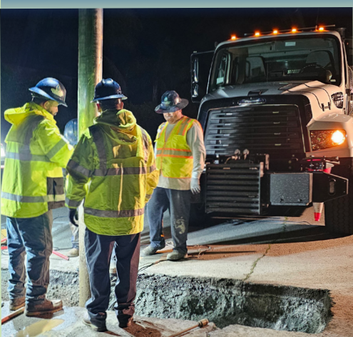
Sunnyslope personnel excavate a pipeline to restore a customer's service after receiving an emergency after-hours call.
